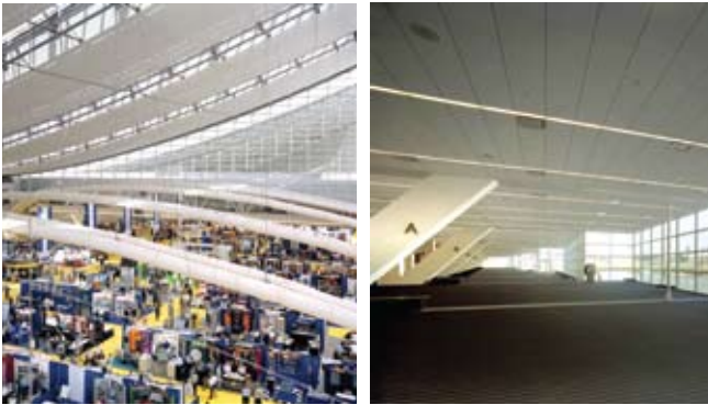
The David L. Lawrence Convention Center in Pittsburgh uses a daylight harvesting system to cut energy consumption by 35%, an annual savings of about $500,000 per year. (Photos courtesy of Leviton)
