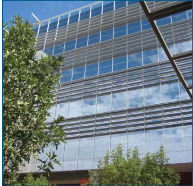
The new Chandler, Arizona City Hall, designed by SmithGroup, was intended to provide effective daylighting, avoiding glare and solar heat gain. (Photo courtesy of SmithGroup)
